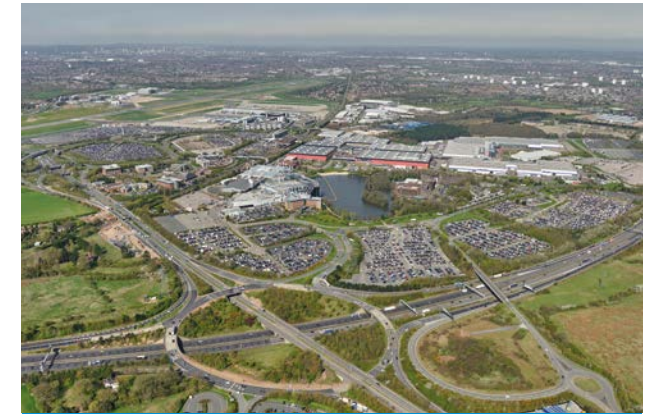
Birmingham Airport sits at the heart of the UK's road and rail networks
