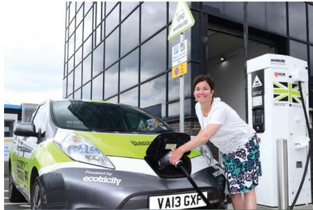
Electric vehicle recharging point
