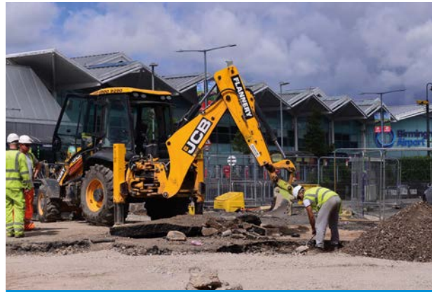
Construction of new Premium Set Down facility was completed in 2017
