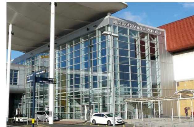
Birmingham International Station and Multi Modal Interchange
